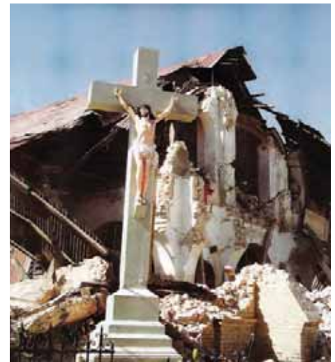
Wreckage of the Port Au Prince Cathedral
